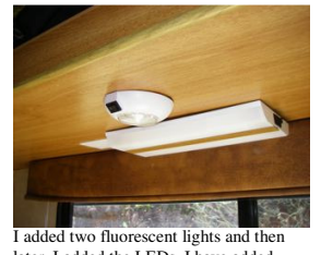
I added two fluorescent lights and then later, I added the LEDs, I have added another since this photo was taken.
