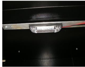
I removed the vent fan as it did not vent to the outside and installed a six light led.
