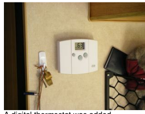
A digital thermostat was added.
